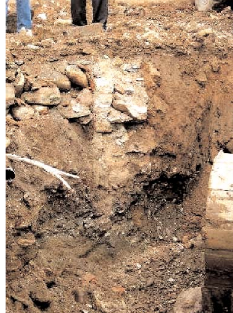
Fig. 26 A building site at Marash. The section of the pit shows the remains of the river stone foundations of the demolished building, and an earlier wall next to it.
