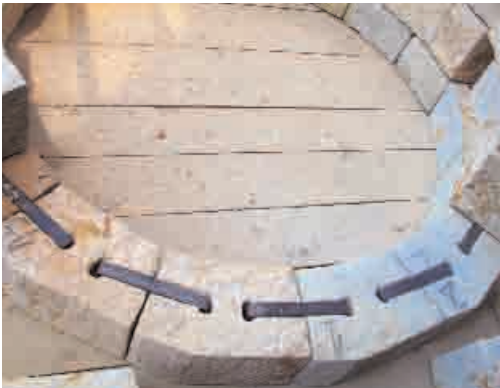
Minaret shaft stones bound with iron clamps
