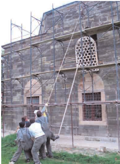
Replacement of iron shutters with white cement grid
