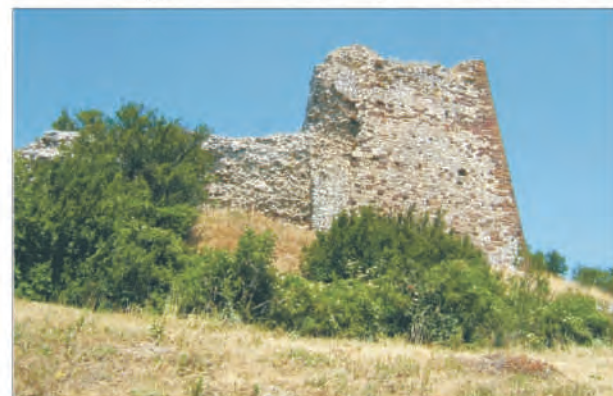
Fig. 22 The southern tower of the Lower Fort in the early 1950s, before conservation works were carried out at its base (after Zdravković 1956, fig. 7), and in 2008.
