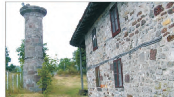
Fig. 35 Novobërda mosque. A view of the patchwork of stone types used as building material.
