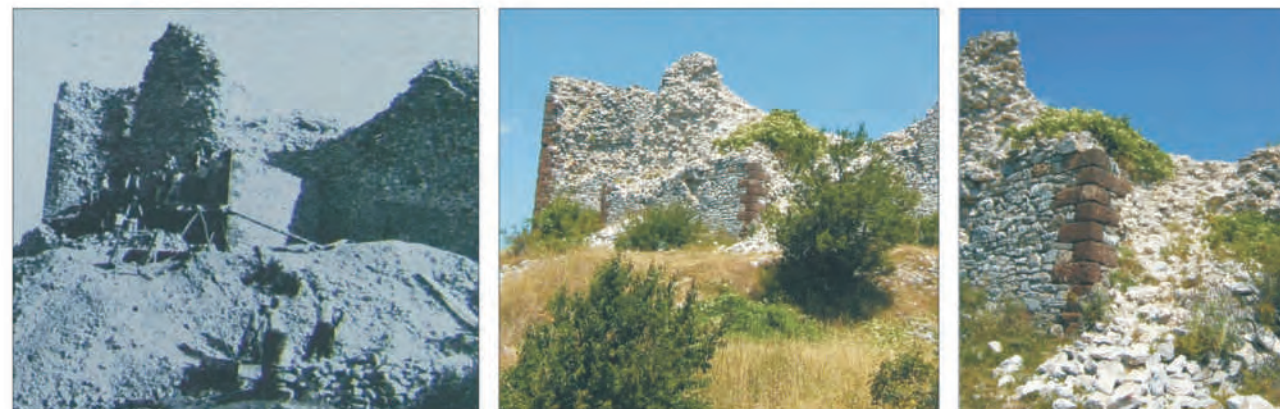
Fig. 24 Tower 3 of the Upper Fort during conservation works (left, after Zdravković 1956, fig. 47), and in 2008.
