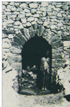
Fig. 20 The entrance between Towers 3 and 4 during excavation, viewed from outside the Upper Fort. The damage to the wall above the entrance has been repaired. After Zdravković 1956, fig. 31.
