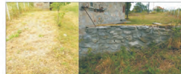
Fig. 38 Novobërda mosque. Left: overgrown feature between the minaret and the mosque. Right: consolidated wall attached to the mosque.
