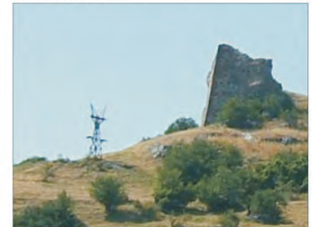
Fig. 47 View of the remains of the "cableway posts" which passes the southern tower of the Lower Fort
