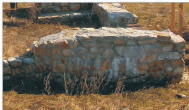
Fig. 34 Restored walls of the Jovan Church.
