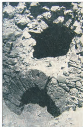
Fig. 19 The entrance between Towers 3 and 4 during excavation, viewed from outside the Upper Fort. After Zdravković 1956, fig. 8.
