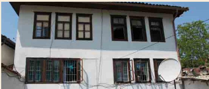
FASADA BALLORE FRONT FACADE
