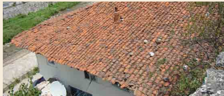
DUKJA E KULMIT VIEW OF THE ROOF
