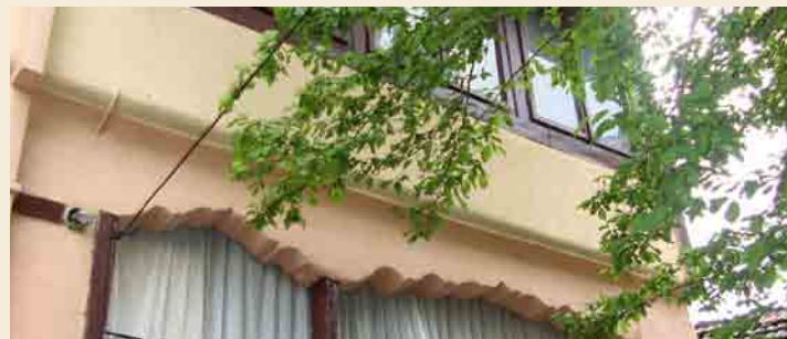
FASADA BALLORE FRONT FACADE
