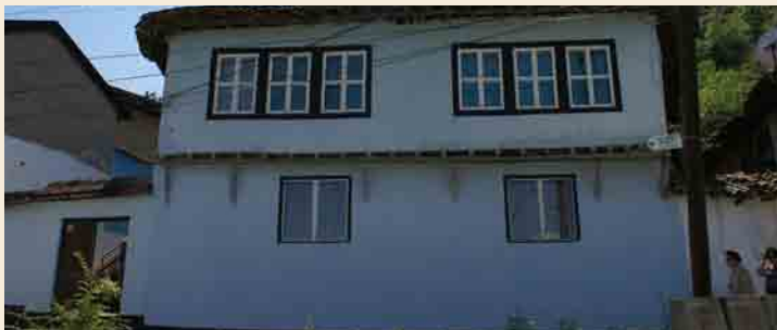
FASADA BALLORE FRONT FACADE
