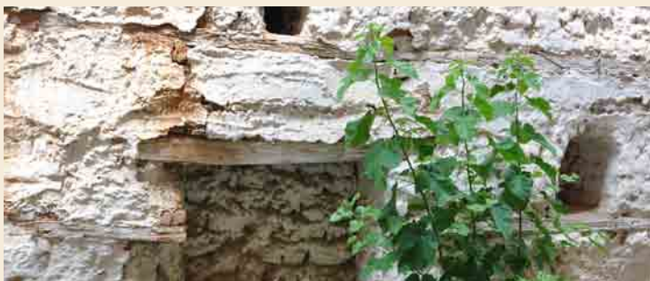
MURI I OBORRIT CONSTRUCTION OF YARD'S WALL
