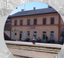
Stacioni i trenit Železnička stanica Train station Viti / Godina / Year: 1873-75
