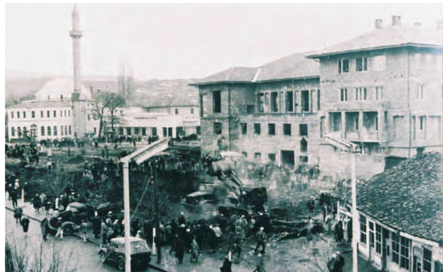
Fig.15 – Pulling down of an old part of the city of Prishtina/Priština
